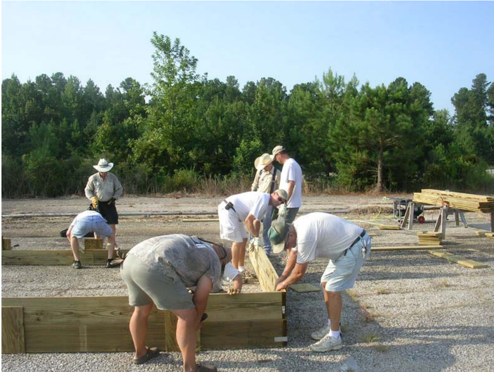
Photo 1: Weevil tank construction
